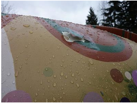
Blister broken and pulled back – no adhesion found
