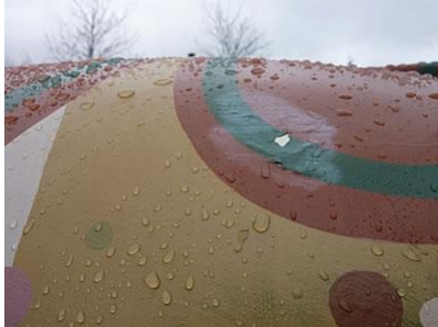
Blister showing delamination of film
