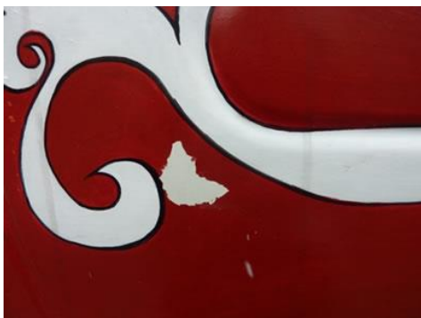
Small delaminated area down to primer
