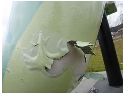
No adhesion of the surrounding paint finish
