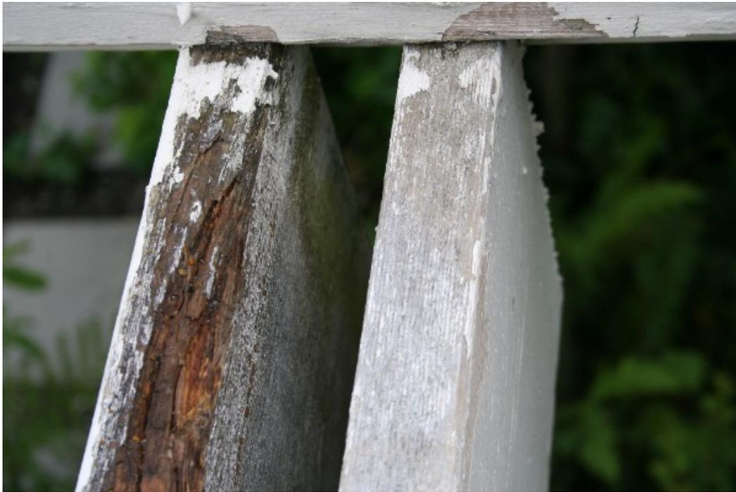
Pictured: Water damage on unprotected wood.
