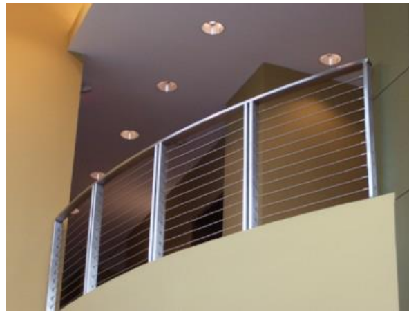
Stainless Steel Handrail
